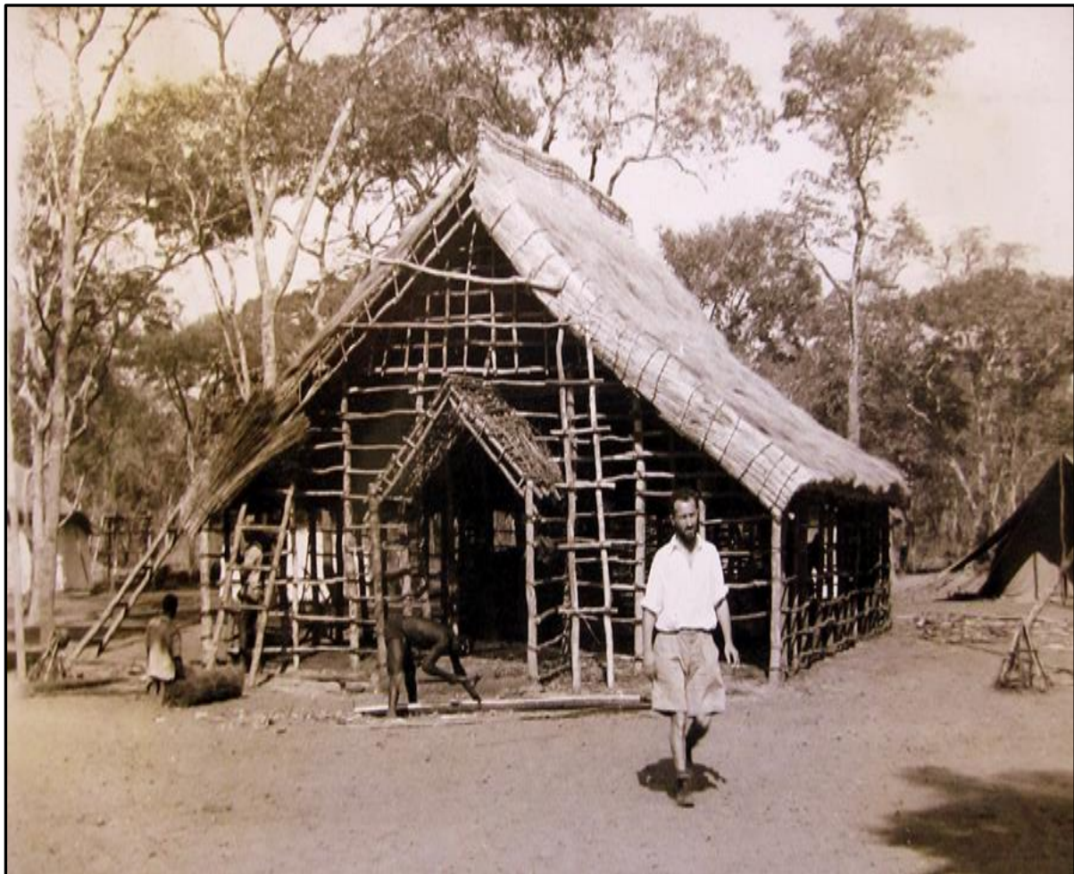
Building a temporary church at the Irish Capuchin mission in Mankoya (now Kaoma), Northern Rhodesia (later Zambia), in 1938. Source: CA/AMI/1/10/1/1
